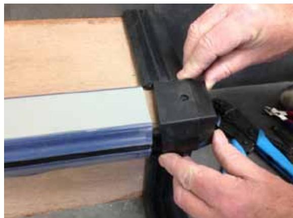
22. Install end cap inserting legs into appropriate retainers.
