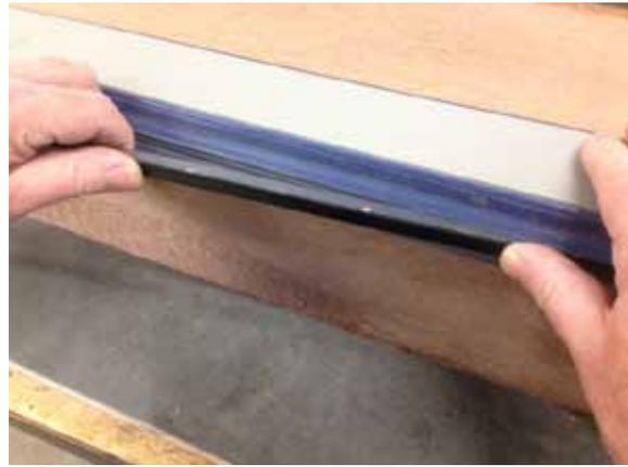
18. Insert tube into stair nosing.
