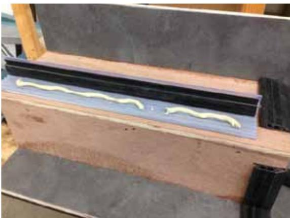
9. Apply adhesive (keeping clear of screw hole & 50mm away from each end).
