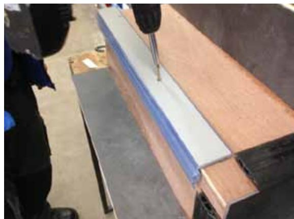
10. Screw nosings (concrete steps require sealant for adhesive to adhere to).
