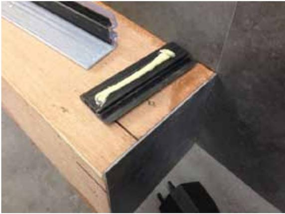
5. Apply gap filling adhesive (Substrate must be in good condition).
